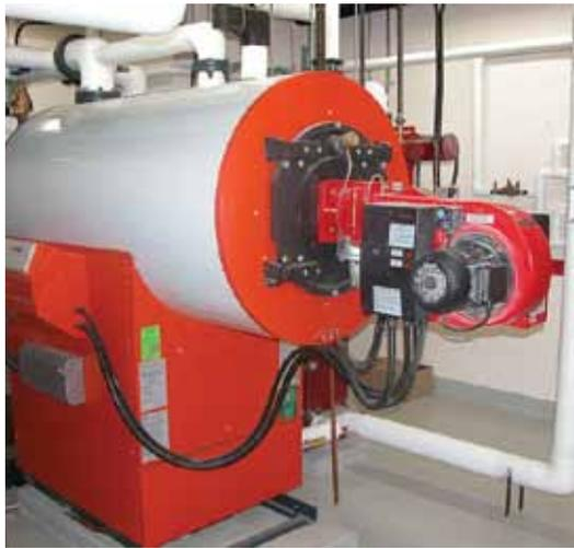
maximise heat transfer from the burner, as well as recovering useful heat which would normally be lost with the flue gases. A condensing boiler will always be more efficient than a conventional non-condensing one, due to its larger heat exchanger.
